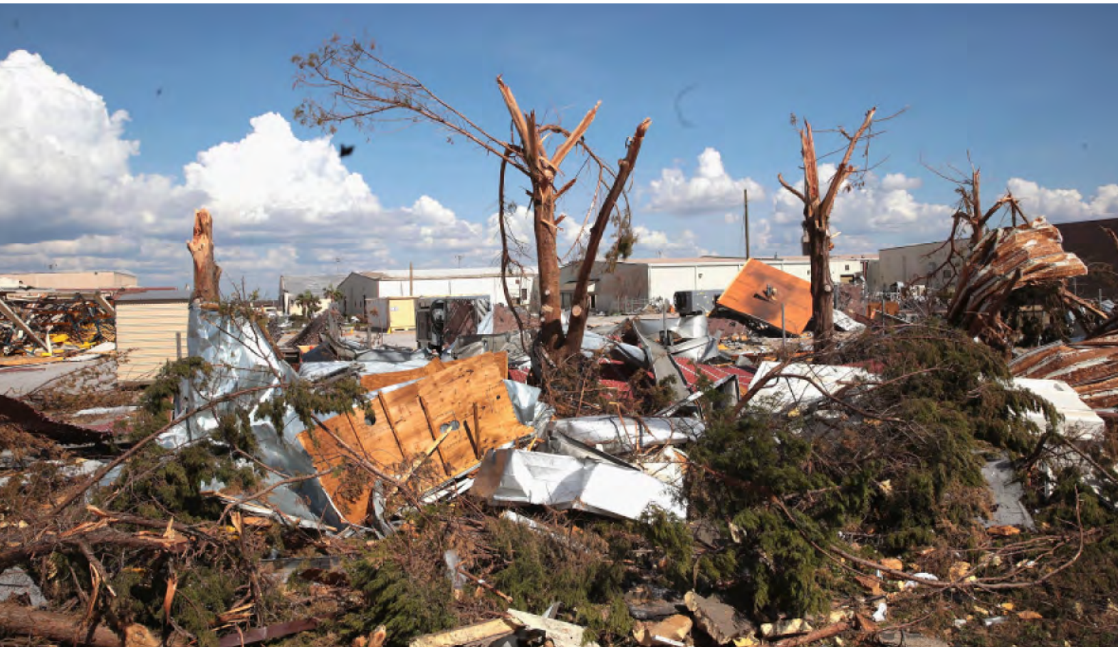
Debris litters Tyndall Air Force Base following Hurricane Michael in October 2018. SCOTT OLSON/GETTY
