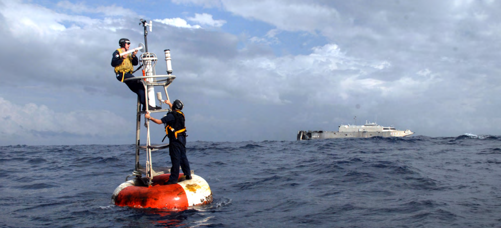
U.S. Navy Minemen 2nd Class Matthew Rishovd and Kody Egelhoff repair a National Oceanic and Atmospheric Administration buoy. U.S. DEPARTMENT OF DEFENSE
